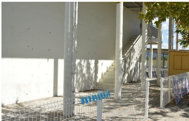
Driving stand stairs
