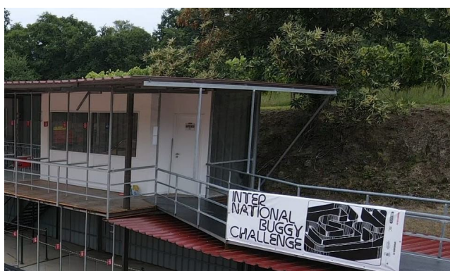
Driving Stand Stairs
