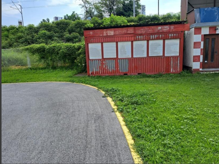
TIME KEEPING ROOM (currently under renovation)
